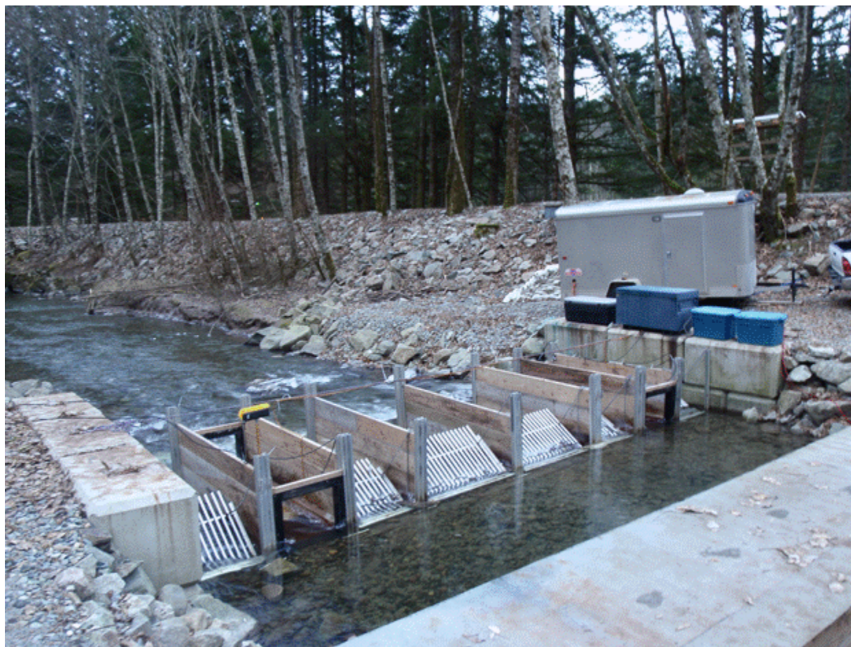
Figure 4. Downstream photo of the NVOS enumeration site showing the design used from 2008-2015 with two channels containing one resistivity counter pad in the centre and two directional antennas (one upstream and one downstream).
