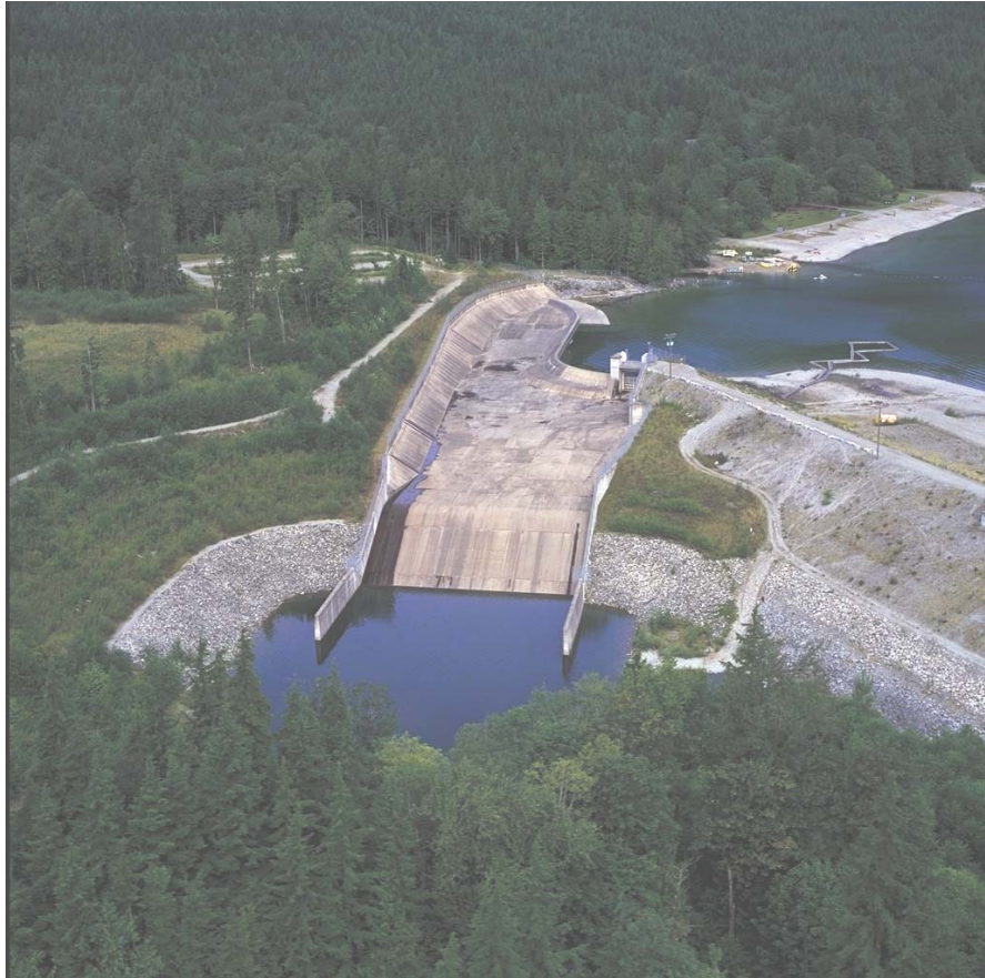
Figure 2-2: Photo of Alouette Dam Spillway
