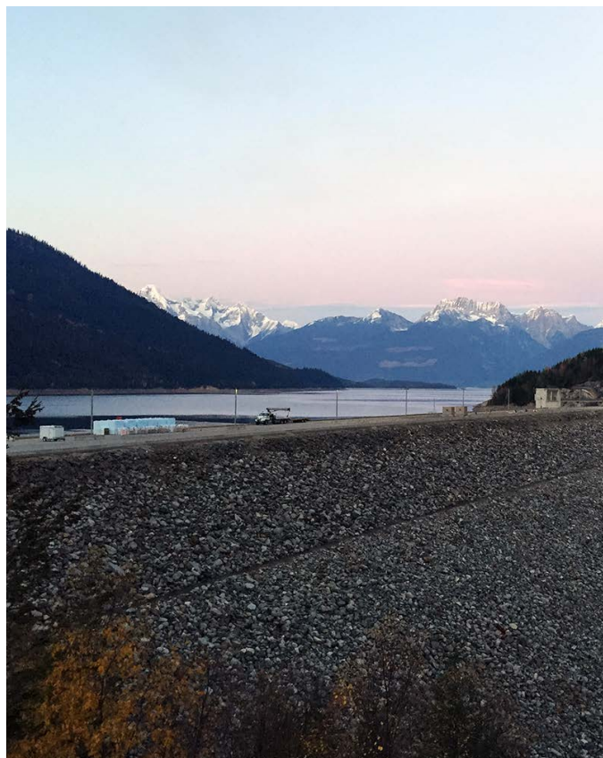
Mica Dam and Generating Station.
